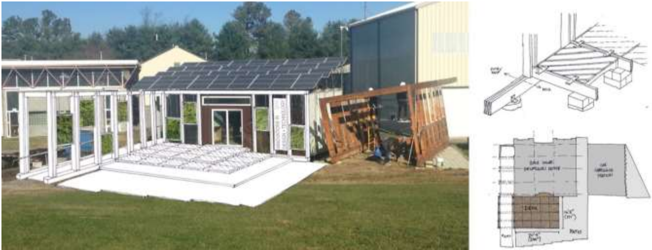
Figure 4: Above: proposal for exterior renovation; middle: deck construction detail; bottom: layout diagram
