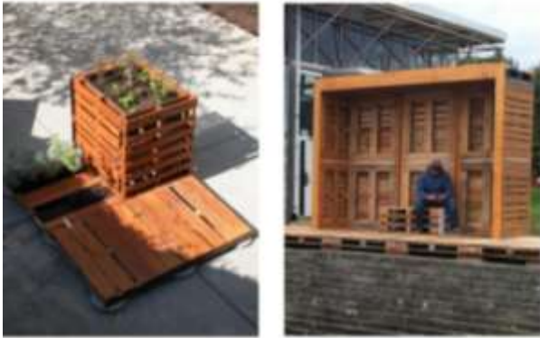
Fig. 1: Left: prototype of the deck and planter; Right: the proof of concept for the pallet wall section
